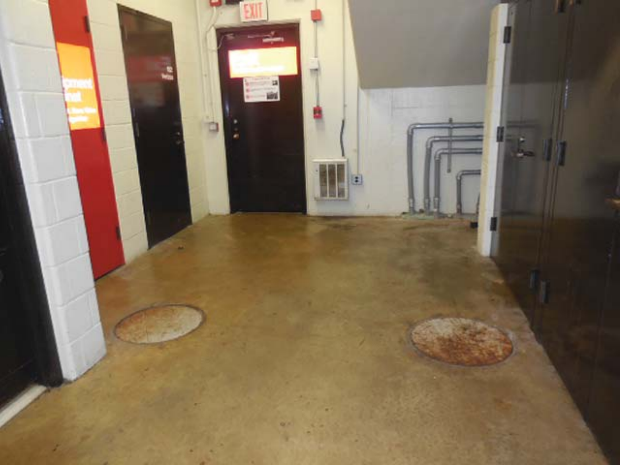
Picture 3: F09 Naylor – Manholes in passageway to Room 126
