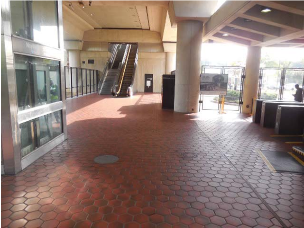
Picture 2: F09 Naylor – Handhole and manhole in mezzanine
