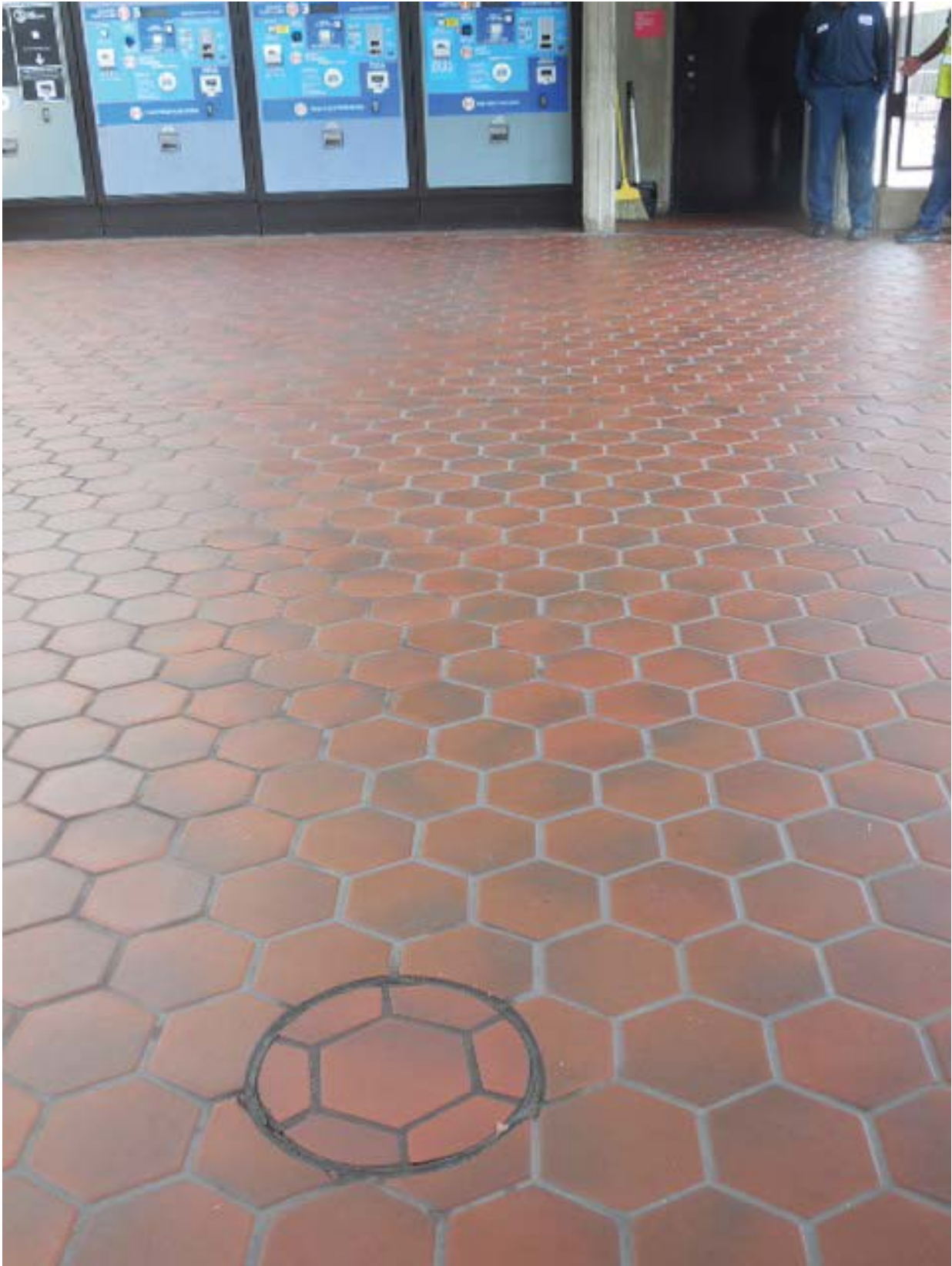
Picture 1: F11 Branch Ave. – Handhole in Mezzanine
